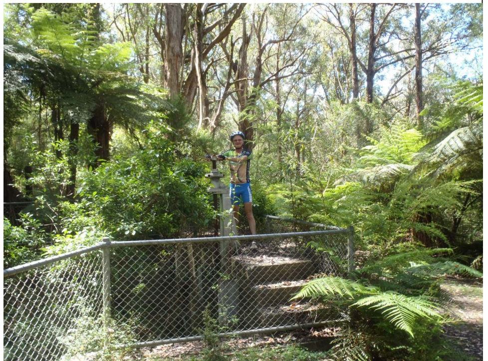
Jeff on one of the remaining control structures on the old O'Shanassy aqueduct.
