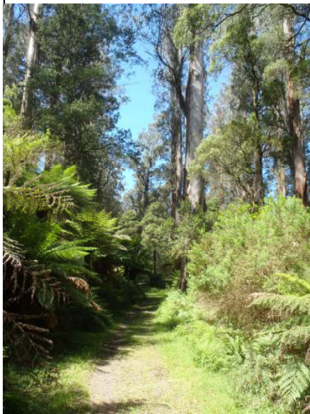
Where has the aqueduct gone? It is hidden in the forest overgrowth in the lower left hand side of the photo.
